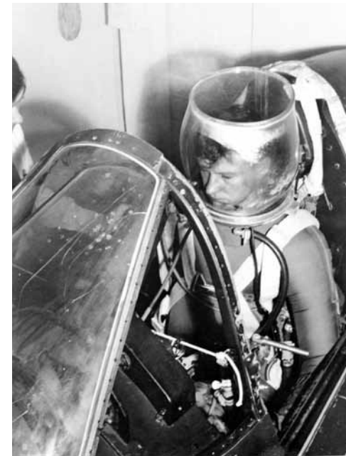
The Experiment B suit in the cockpit of a Vought F4U the Navy had loaned David Clark Company during July 1949. One of the major failings of the Experiment B suit, and most early pressure suits, was a lack of ventilation that caused the wearer to perspire excessively.
